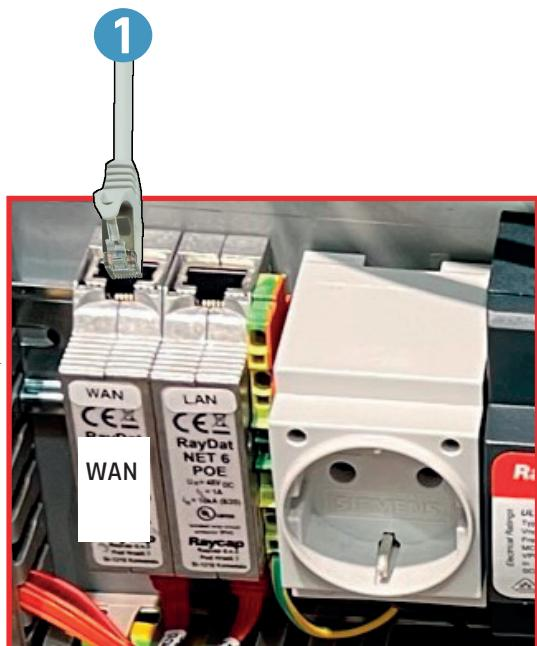
Fig. 31: Connection of communication ECC 320
