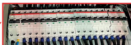
Fig. 23: Line/fault-current circuit breakers
