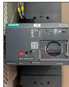
Fig. 55: Motorized switch disconnector
