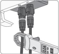
9 Disconnecting the Inverter from Voltage Sources
